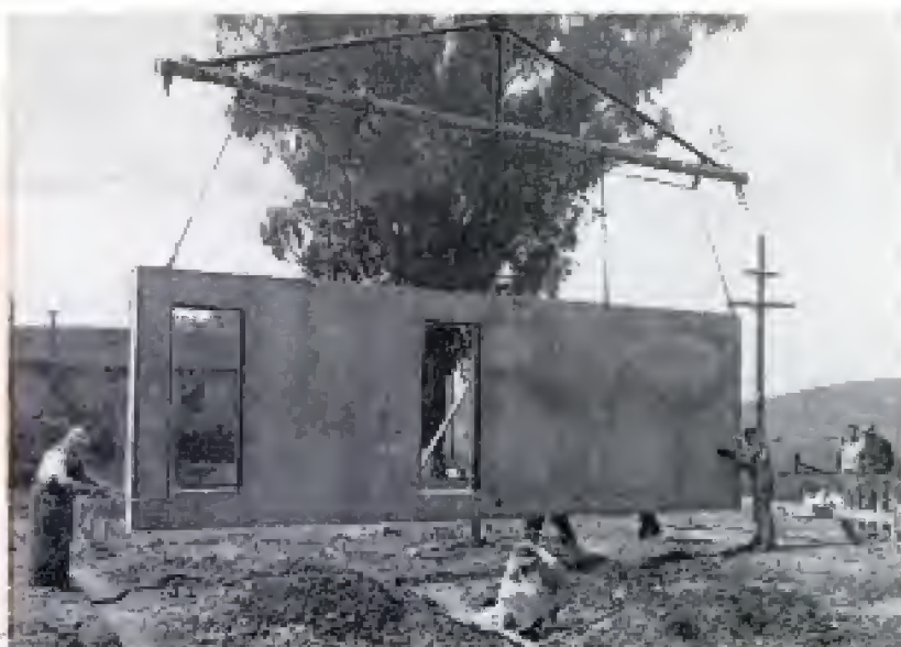
Workmen prepare to guide one-piece wall section into place. The wall is six inches thick and made of steel-reinforced lightweight concrete. The door and window frames are cast right into the solid wall.
